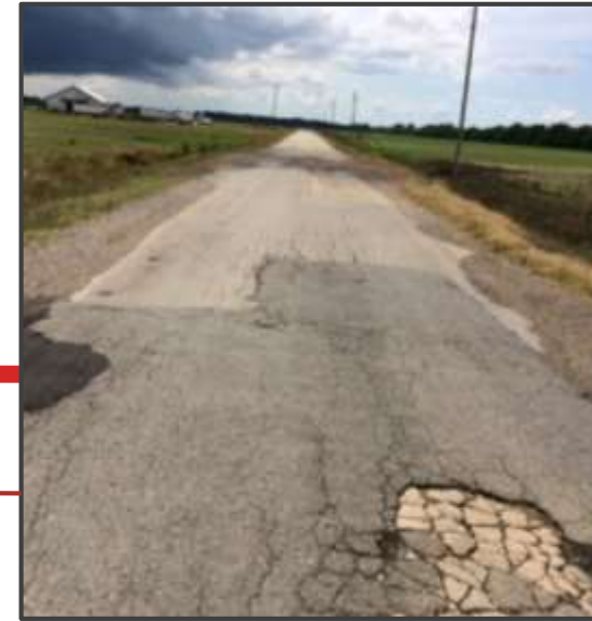
Chicot County, Highway 144 Lake Chicot State Park entrance to the Mississippi River Levee
